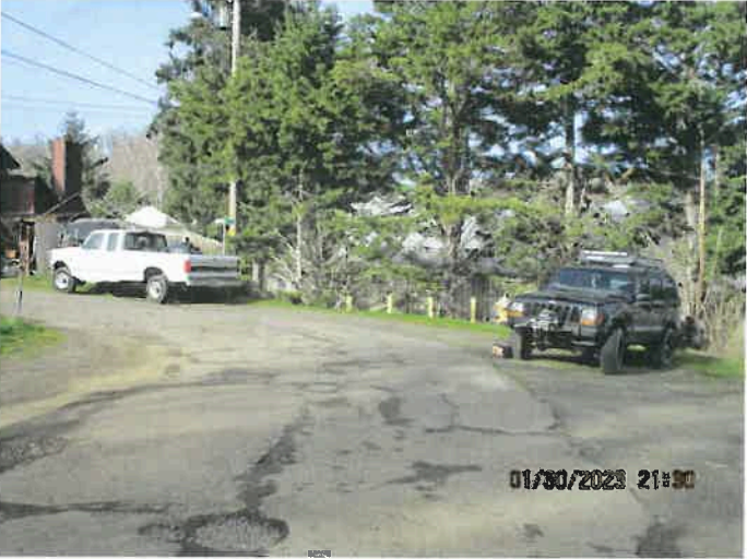
Fire hydrant boat & car park on NW Merle (2)
