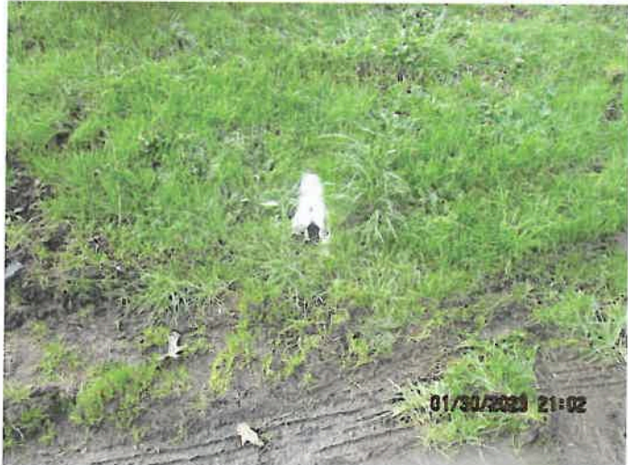
1780 NW Merle drain pipe 1 (1)
