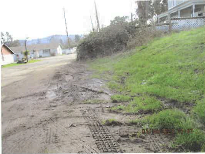
1780 NW Merle drain pipe 1 (2)
