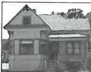
Queen Anne style homes have multiple roof forms such as this combination gable and hip roof with bay window
