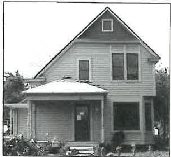
The historic character and street appeal are restored after rehabilitation of the siding, reconstruction of the trim and repainting
