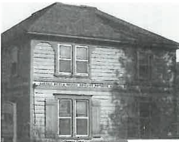
Original 1/1 double-hung windows and details
