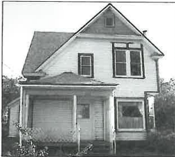
During rehabilitation, the incompatible metal siding was removed, and original wood siding exposed and restored. Paint lines indicate location of original trim
