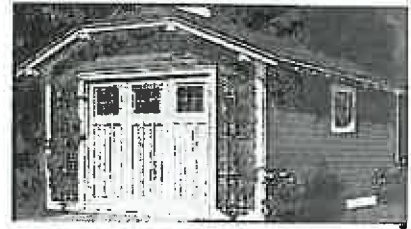
Examples of garages built in the early 1900s from Sear Roebuck & Co. catalogue. Refer to historic examples in designing new garages
