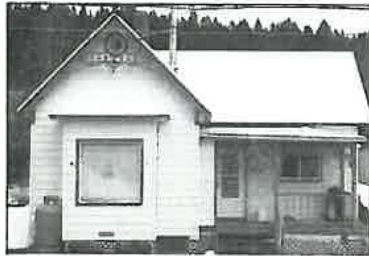
Vernacular Queen Anne cottage with incompatible new picture window and aluminum slider
