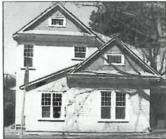
Height and Scale: The addition (left) on the Queen Anne cottage is too high and out of scale with the house. Although consideration was given to applying compatible design elements, the original house becomes "lost"
