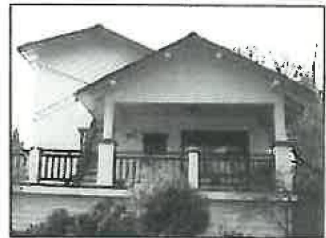
Scale and Materials: Although setback, the two-story addition (left) is not compatible with the scale, height, proportions, or materials (diagonal siding) of the Bungalow style house.
