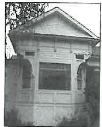
Excellent example of a Victorian era house in Mill-Pine that has a variety of siding materials applied as decoration
