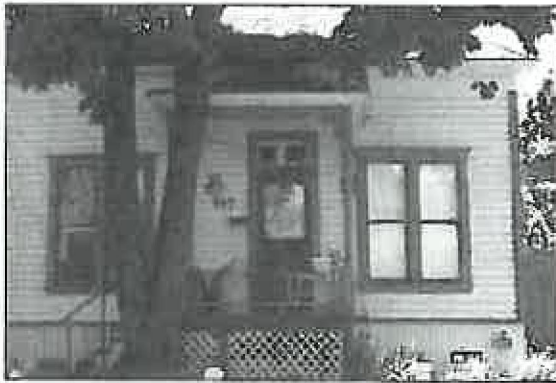
Original window and door types common in the District; paired, 1/1, double-hung wood sash windows
