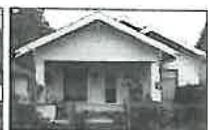
Bungalows generally have low to moderately pitched gable roofs supported by brackets.
