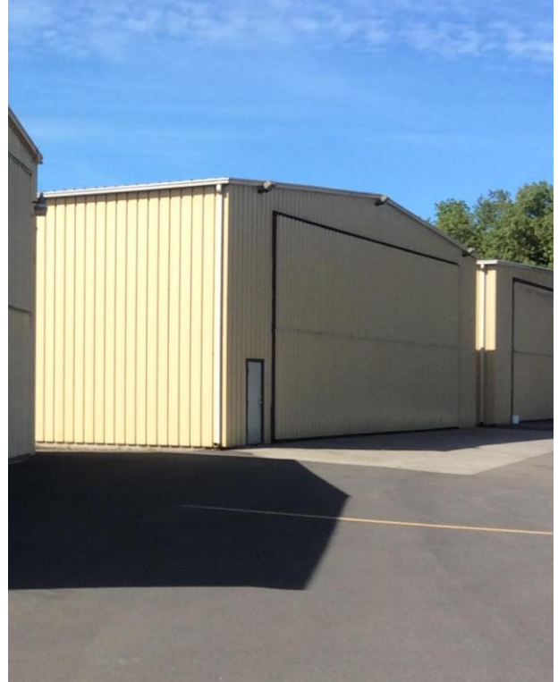
Figure B-29. Building 2381
