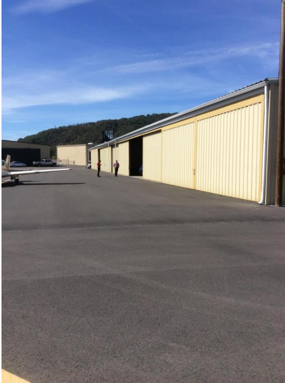
Figure B-14. E-Hangar
