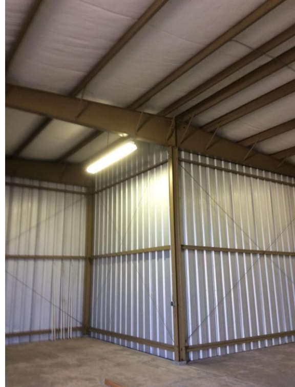
Figure B-13. D-Hangar
