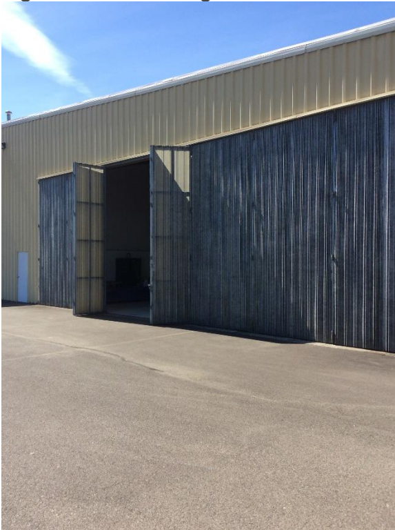
Figure B-6. Lear Hangar
