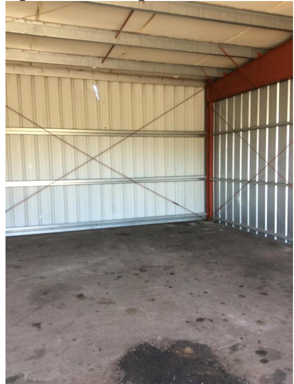
Figure B-11. C-Hangar
