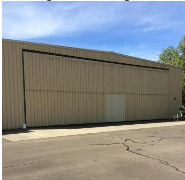
Figure B-30. Building 2391
