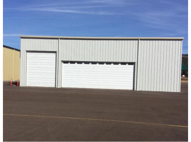
Figure B-39. Building 2777
