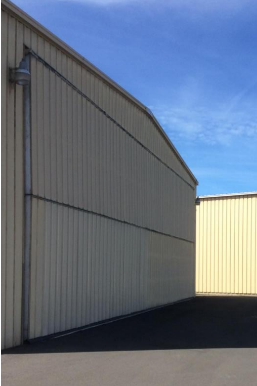
Figure B-28. Building 2371
