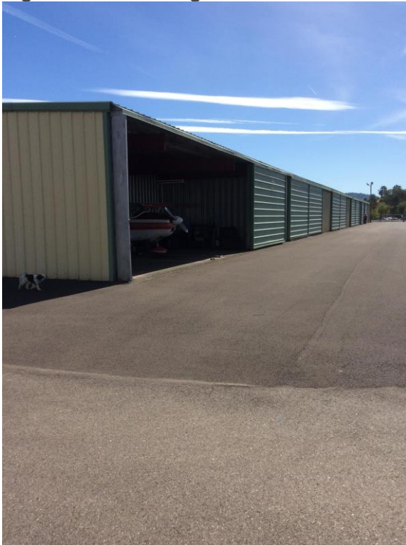
Figure B-10. C-Hangar
