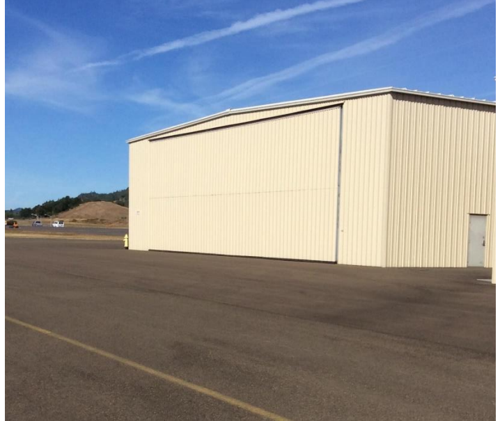
Figure B-42. Building 2815
