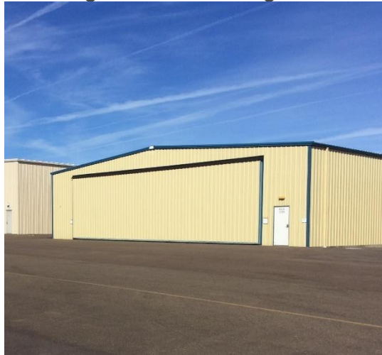
Figure B-40. Building 2785
