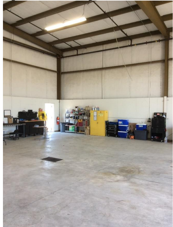
Figure B-7. Lear Hangar
