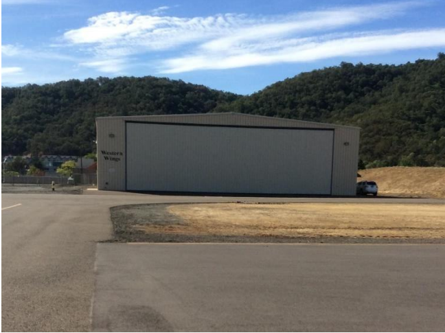
Figure B-38. Building 2825
