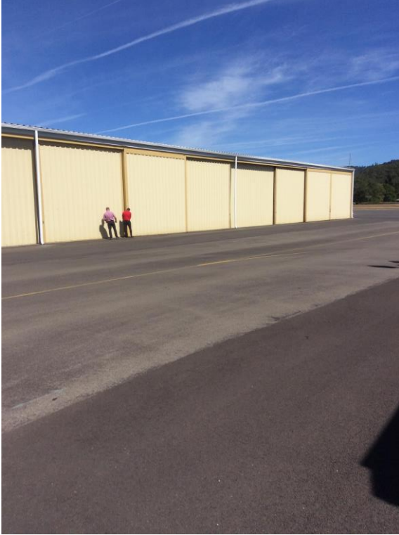
Figure B-12. D-Hangar
