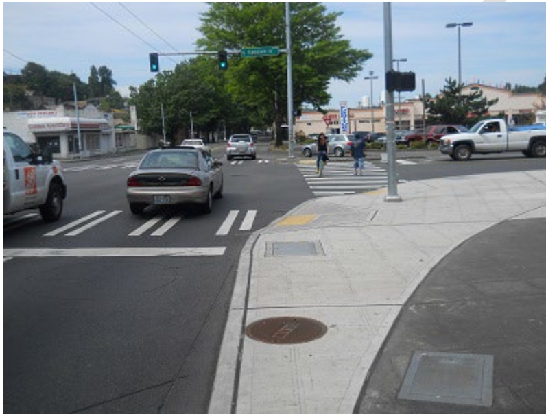
Photograph 3. Redesigned Curb with Reduced Turning Radius – Maricopa Association of Governments (azmag.gov)
