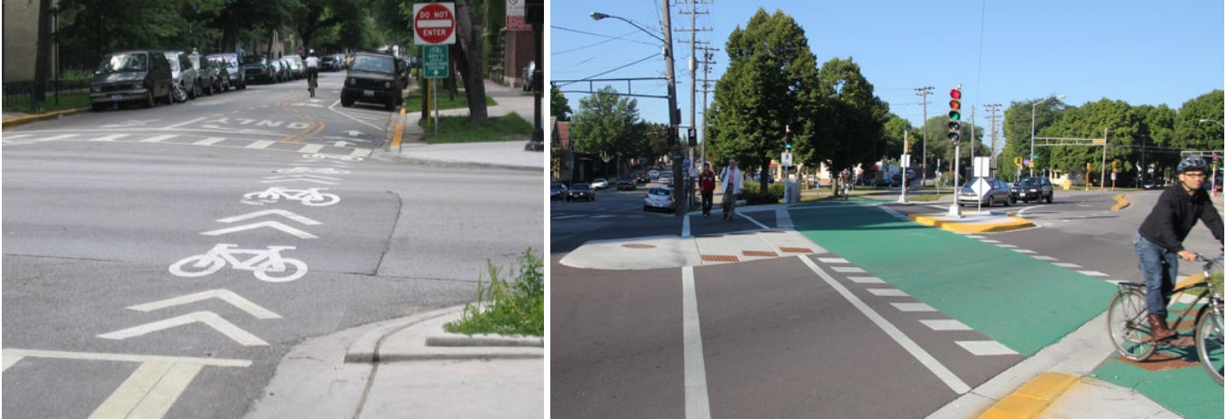
Photograph 5. Intersection Crossing Markings – NACTO Urban Bikeway Design Guide
