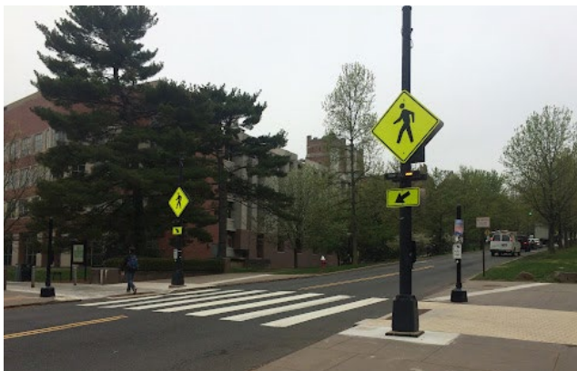
Rectangular Rapid Flashing Beacon – Pedsafe (pedbikesafe.org)
