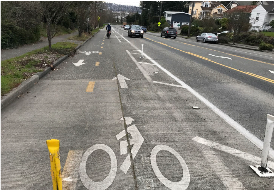
Figure 2. Two-Way Separated Bike Lane with Flexible Delineators in Seattle
