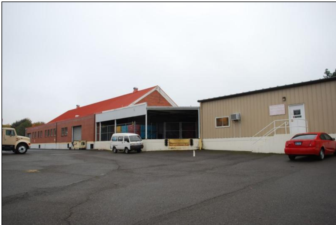
Photo 16 of 16: View looking to the east-southeast along the façade (northwest elevation) of Resource 11 and 11A.
