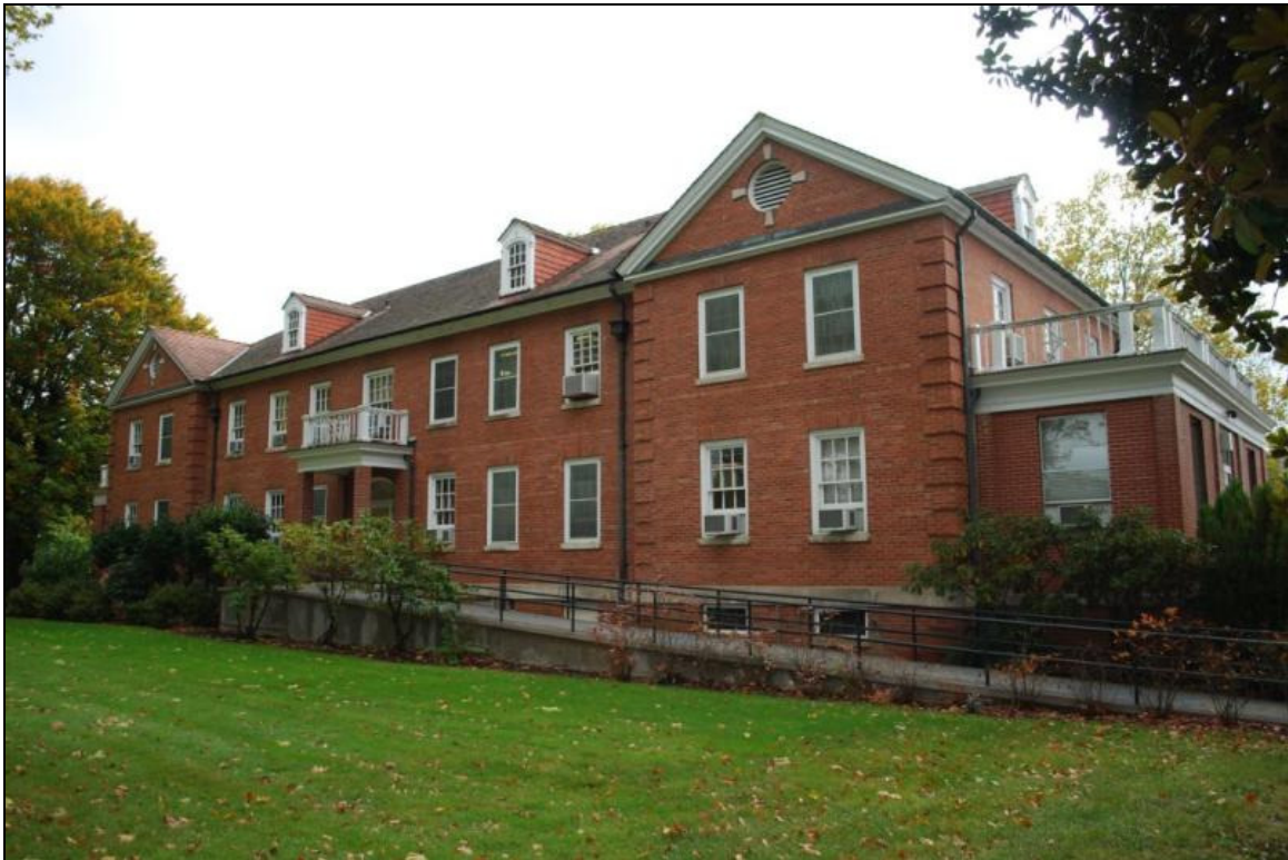
Photo 12 of 16: Façade (northeast) and northwest elevations of Resource 3. View looking south-southeast.
