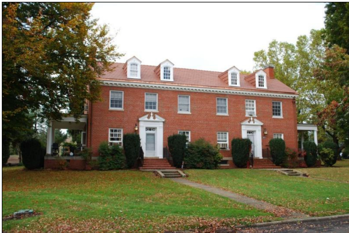
Photo 10 of 16: Façade (southeast) elevation of Resource 6. View looking north-northeast.
