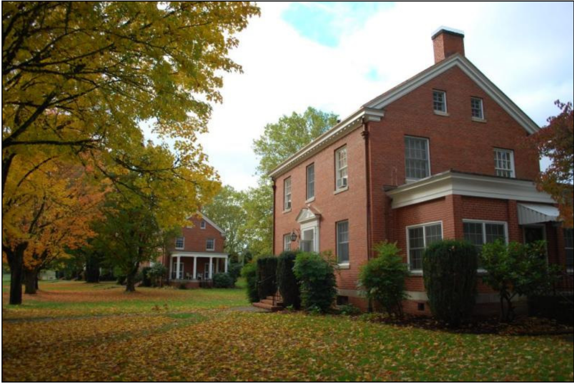
Photo 11 of 16: Façades (southeast) and northeast elevations of Resources 5 and 6. View looking southwest.
