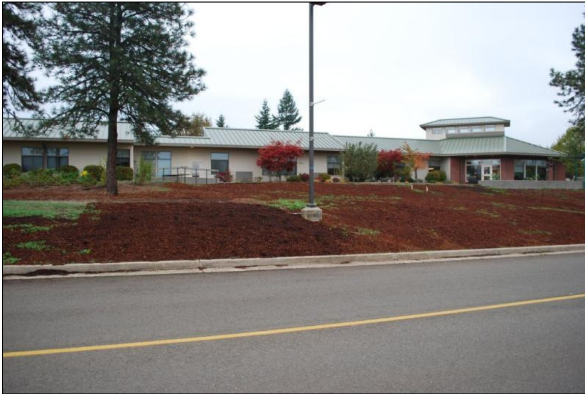
Photo 9 of 16: West elevation of Resource 81. View looking east-southeast.
