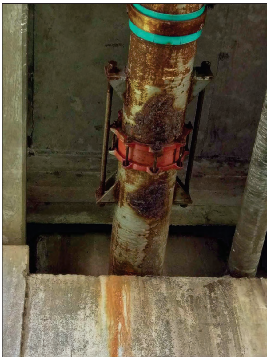
PHOTO 1 - WATER PIPE COUPLING
