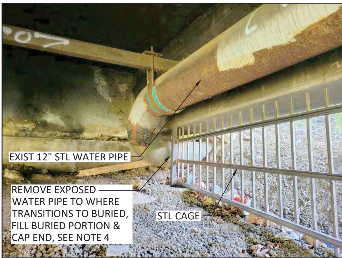
PHOTO 3 - WATER PIPE INTO BRIDGE ABUTMENT
