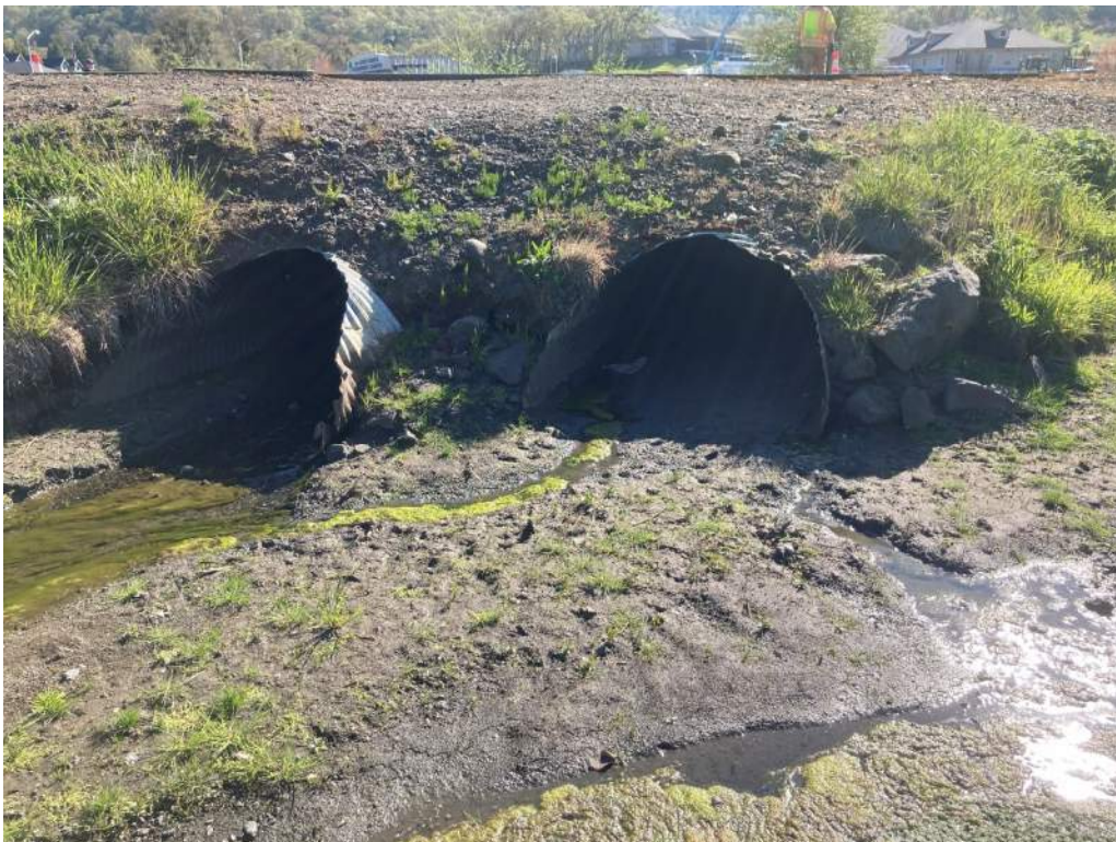
Photo 2. Existing CMP culverts.
